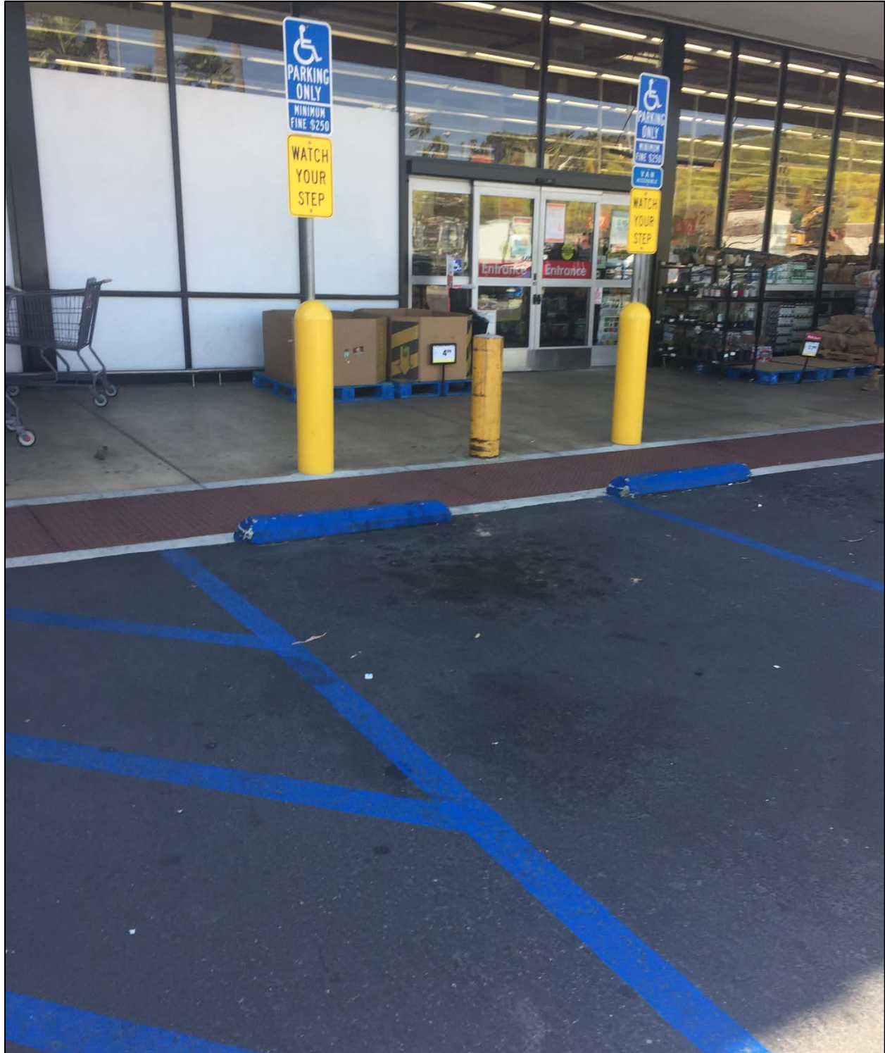
Photo 4 – At this busy storefront in Southern California, multiple pedestrian customers suffered trip-and-fall injuries at these non-required and unnecessary wheel stops.
