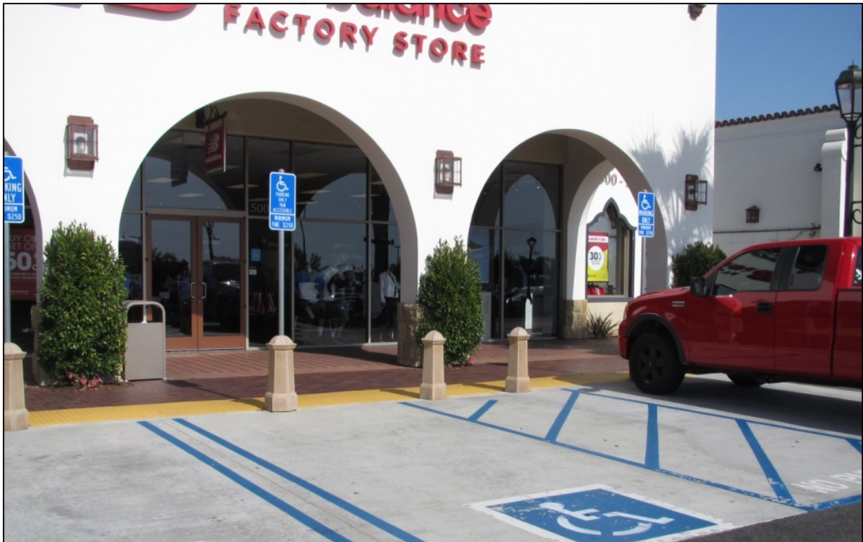
Photo 5 – Structural bollards prevent vehicular encroachment into the accessible route of pedestrian travel.
