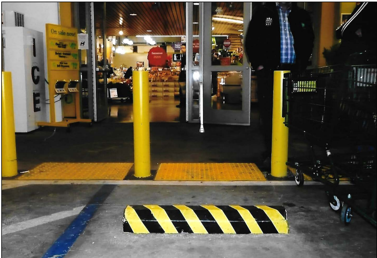
Photo 14 – Case Study #1: after multiple pedestrian falls, this dangerous, non-required wheel stop was removed.
