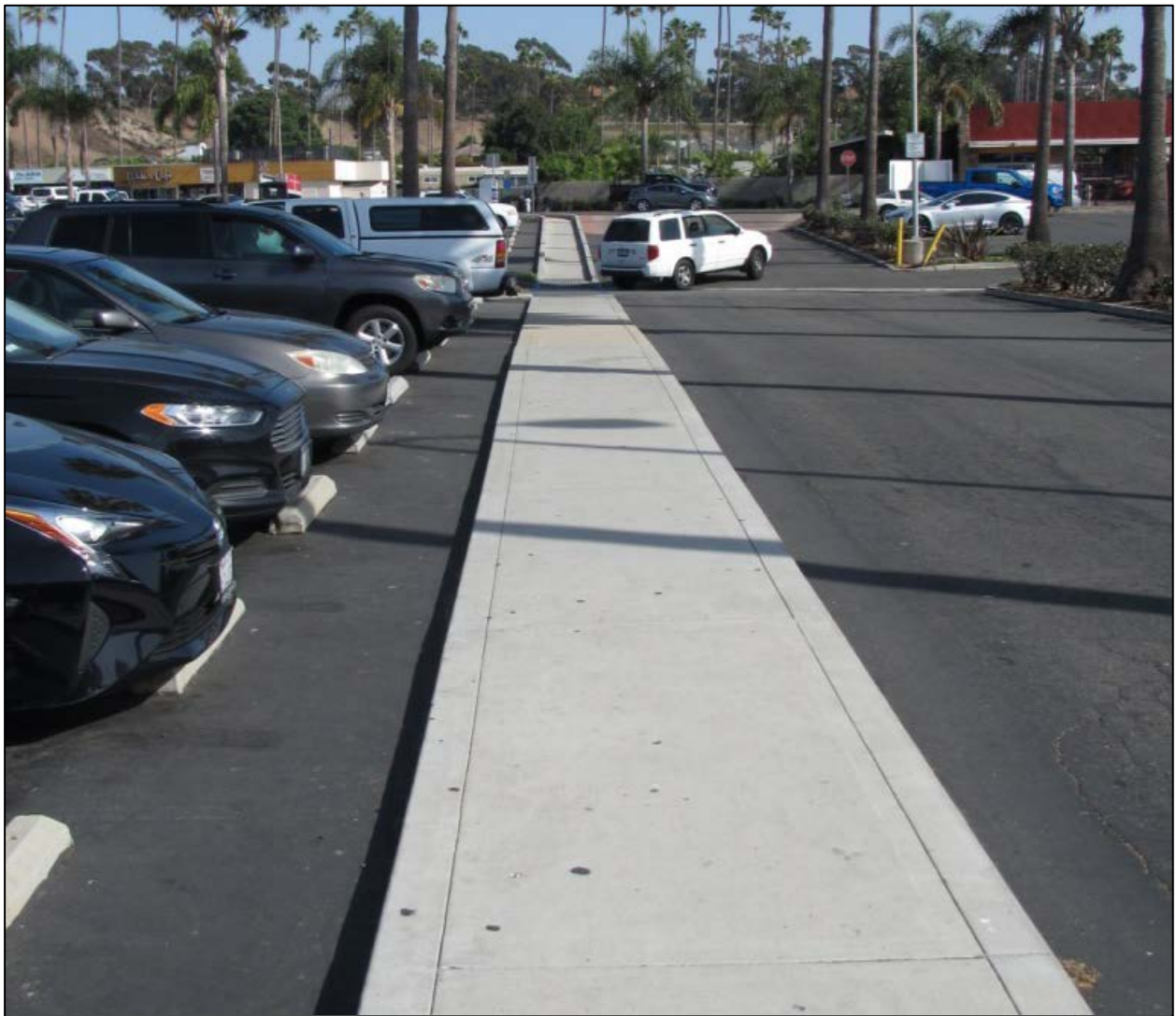
Photo 3 – At this shopping mall in Southern California, the concrete wheel stops deter vehicle encroachment into the required clear width (60 inches) of this wheelchair-accessible sidewalk.
