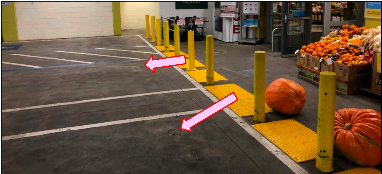
Photo 16 – Case Study #1: after multiple falls, these dangerous, non-required wheel stops were removed.
