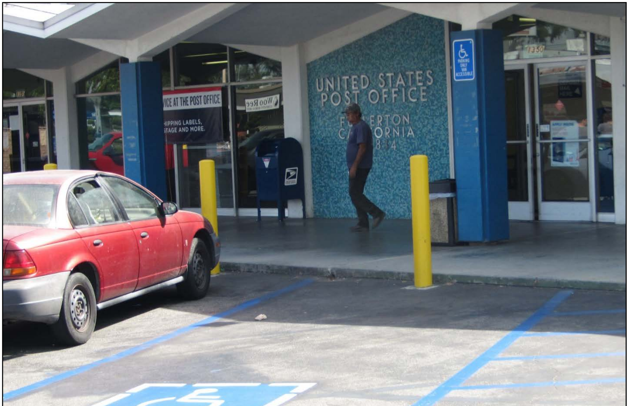
Photo 2 – Similarly, in this parking lot serving a U.S. Post Office branch in Fullerton, CA, original wheel stops have been replaced with structural bollards to better protect customers and employees.
