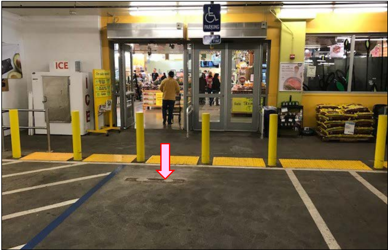
Photo 15 – Case Study #1: after multiple pedestrian falls, this dangerous, non-required wheel stop was removed.
